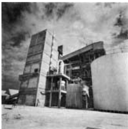
Specialized scrubber system at Monomeros Colombo Venezolanos plant in Barranquilla, Colombia.
